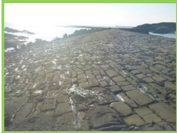
Cullercoates North Pier – sloping seaward face (4701C07)
