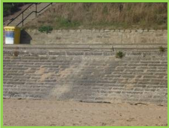
Sloping blockwork revetment (/4701C19)
