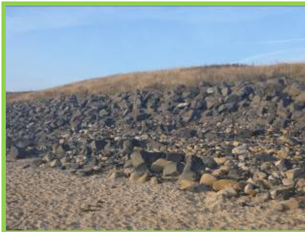
Rock revetment near Briardene Burn (/4501C06)
