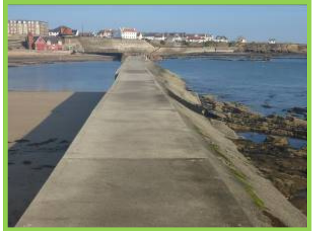
Cullercoates South Pier – deck and sloping seaward face (/4701C15)
