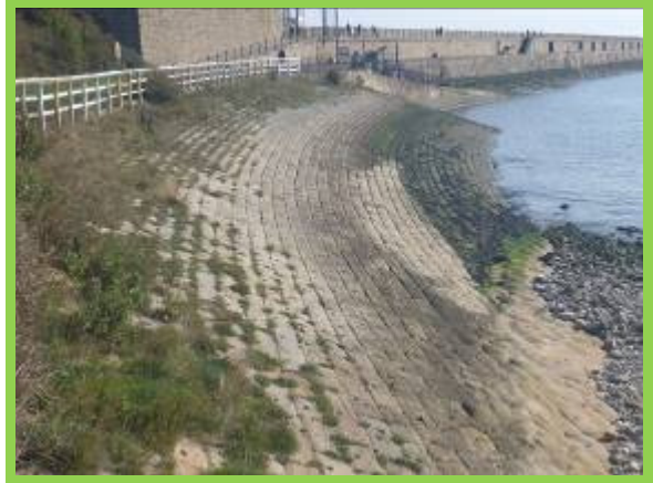
Masonry revetment (/4801C02)
