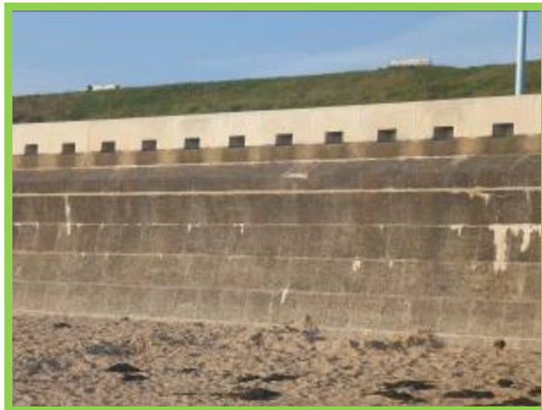
New coping on blockwork seawall (/4501C08)
