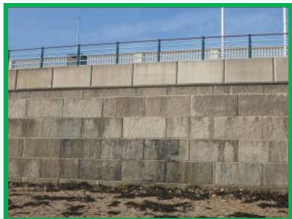
Refurbished sea wall (typical of /4601C02 and /4601C03)
