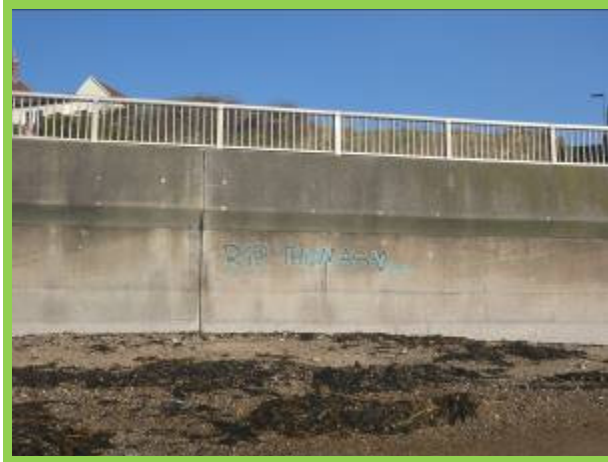
First section of sea wall in generally good condition (/4701C04)
