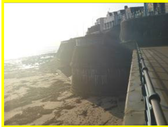
Blockwork sea wall at first 'bullnose' (/4601C04)
