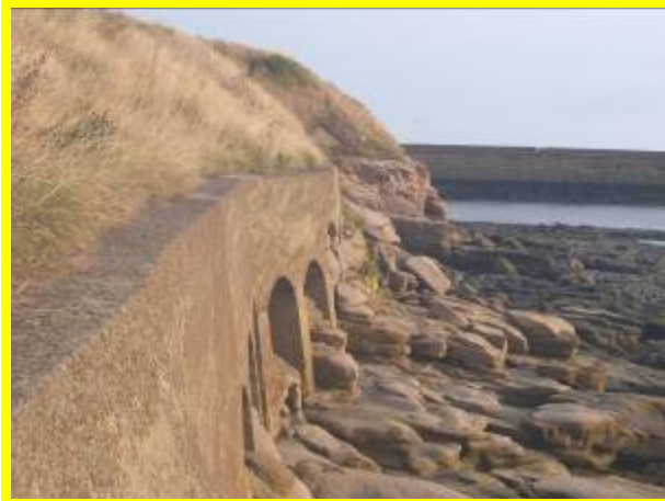
Masonry and concrete arched seawall (/4801C04)
