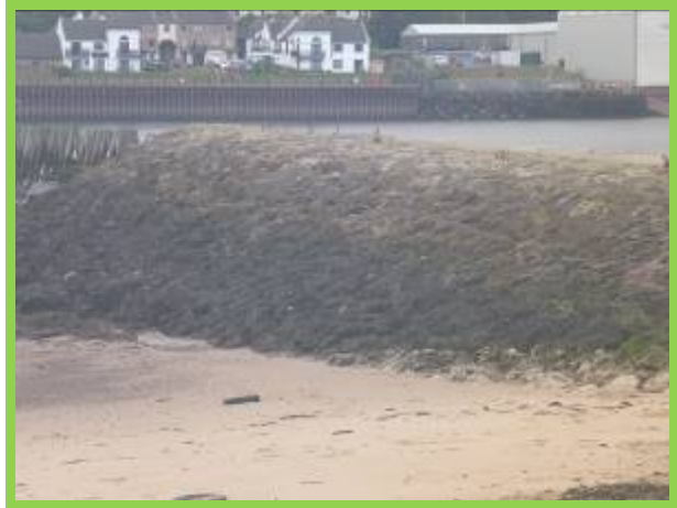
Pitched stone revetment (/4801C10)
