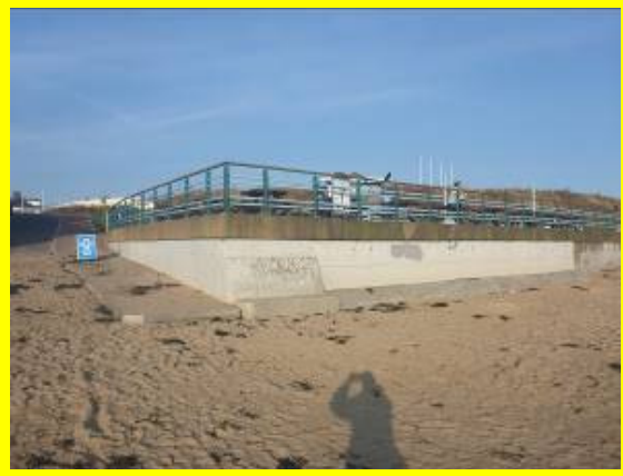
Refurbished seawall at kiosk north of beach access ramp (/4501C09)
