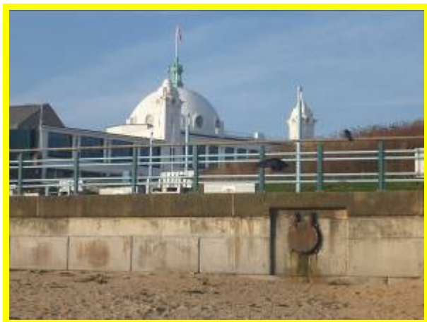
Short section of panel wall (/4501C09)
