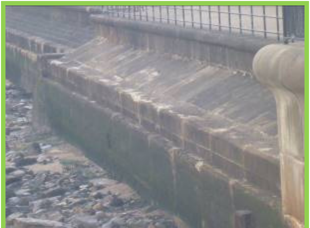
Concrete panel sloping revetment and high concrete toe wall (/4801C08)
