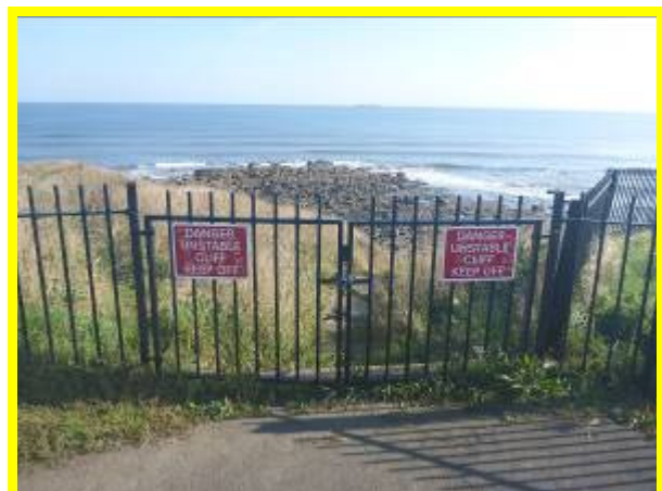
Unsafe access steps now closed-off (/4701C26)
