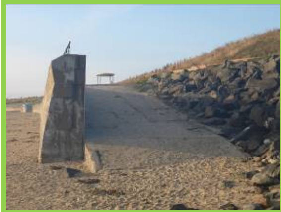
Northern access ramp (/4501C07)
