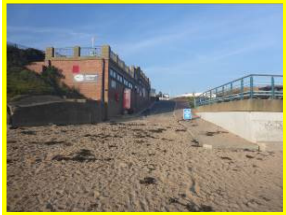
Transition between 4501C09 and 4601C01 at beach access ramp / slipway
