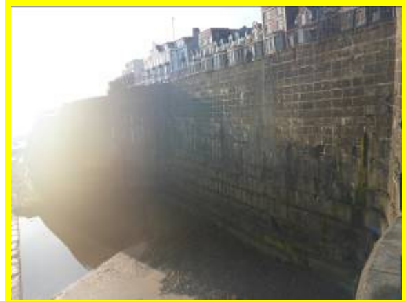
High blockwork sea wall (/4601C04)
