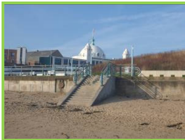
Transition between 4501C08 and 4501C09 at beach access steps
