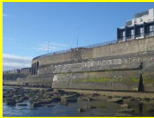
Intermediate sea wall between Central and Southern Promenades (/4601C06) – from 2020 inspection
