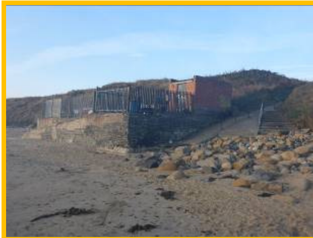
Wall at boatyard (/4501C05)
