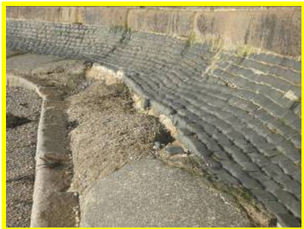
Final section of sea wall in generally fair condition (/4701C06)
