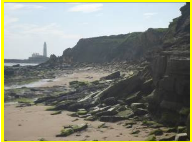
Rock falls in hard material along lower cliffs (/4401C22 & 24)
