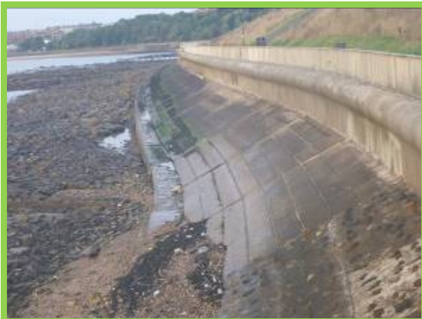
Concrete panel sloping revetment and short concrete toe wall (/4801C07)
