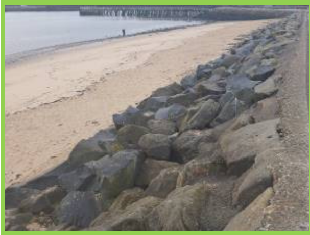
Rock revetment (/4801C09)
