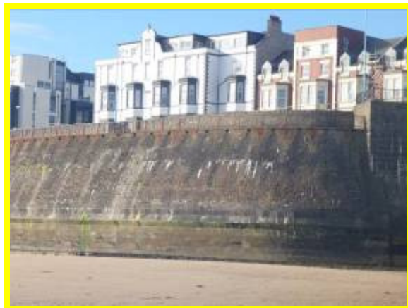
High blockwork sea wall (/4601C05) – from 2020 inspection
