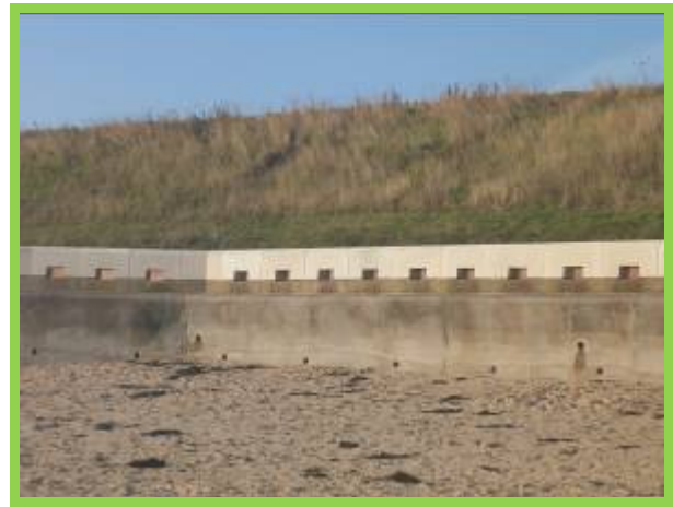
New coping on concrete recurved seawall (/4501C08)
