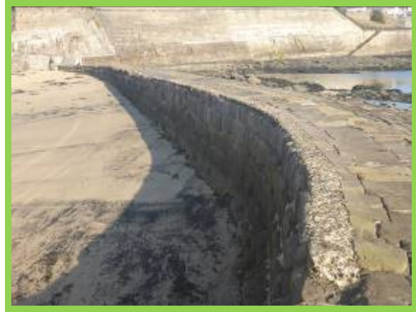
Cullercoates North Pier – deck and vertical landward face (4701C07)
