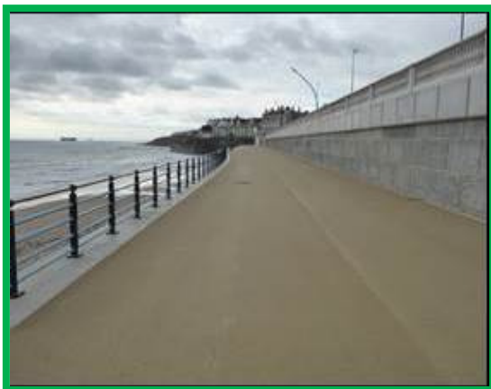
Refurbished promenade (typical of /4601C02 and /4601C03)
